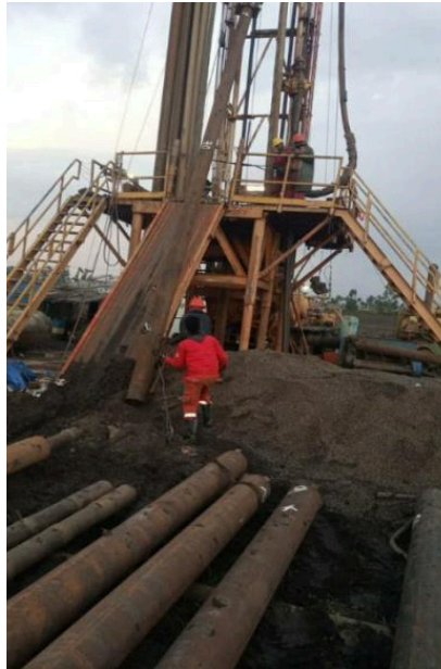
Casing installation at well 5
