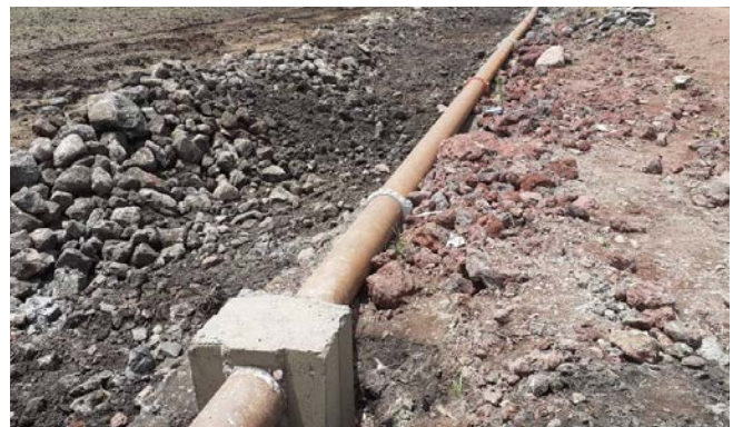
All anchor block works to support pipeline finalized
