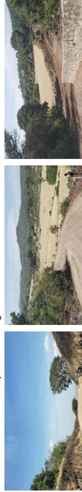
**Access Road** to well pads and reservoir is passable; this is also accessible for heavy load. Finishing works will be done upon completion of Pad GA and water reservoir. Pad GA leveling, compaction and cellar works are almost finalized. OE sent representative to Olkaria to physically see requirements and Kengen has revised the Cellar design.
