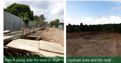
Trench along side the road in Iteya
